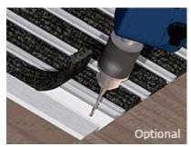
Retire partially or slide the finish strips. Drill the initial and ending profile on both ends to fix **Basmat** to the floor.
